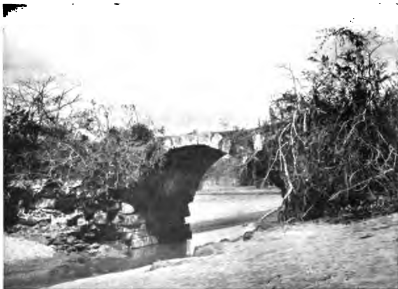
THE BRIDGE LEADING INTO OLD PANAMA.
